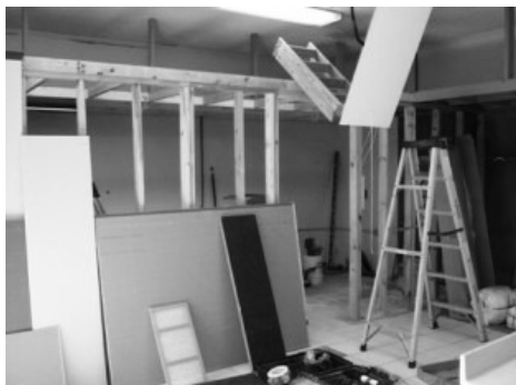
Kids Room During Renovation
