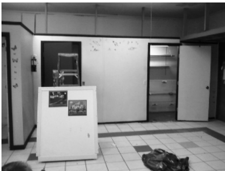
Kids Room Before Renovation
